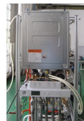
侧面悬挂热水器 Lifting of Gas Water Heater
